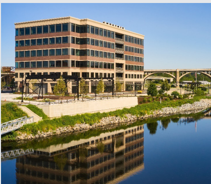
The Waterfront is a $425 million mixed-use development being constructed along the Lehigh River in Allentown.
